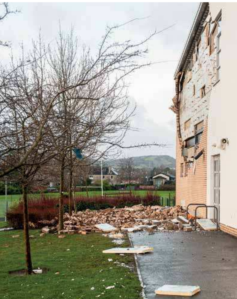
The collapse of the brickwork façade of Oxgangs primary school in Edinburgh in March 2016.
